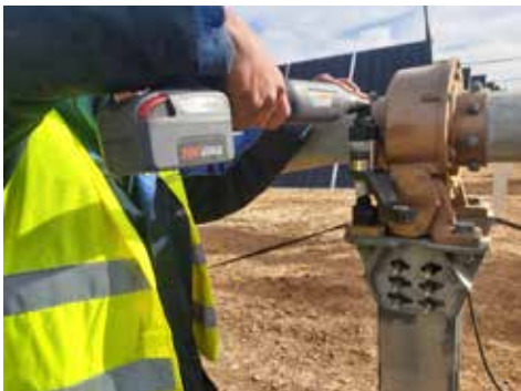
150Nm – 500 Nm bolt tightening
