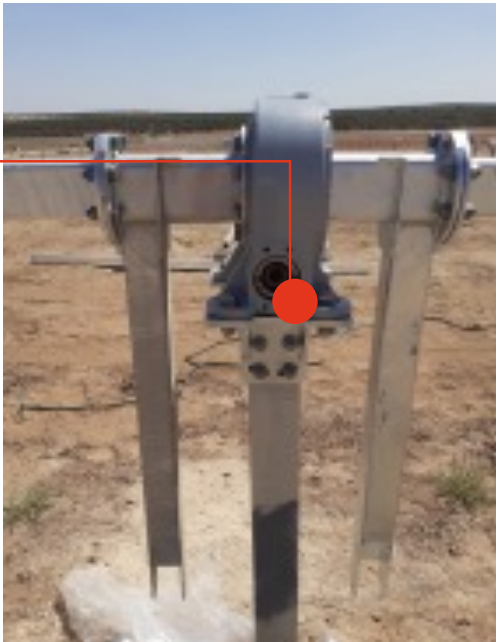
150Nm – 500 Nm bolt tightening
