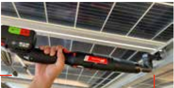
18-21 Nm bolt tightening
